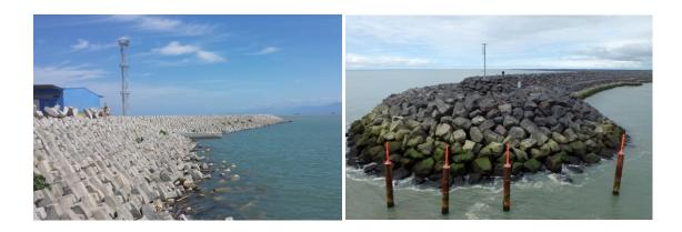
Figure 4. Breakwater structures that exclude penguins include those with very large blocks, and with no crevasses suitable for penguins to roost or breed in. Little penguins are too small to climb structures like these, pictured. Images: Van der Meer Consulting (2017).
